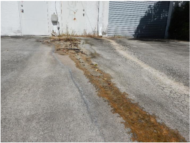
Photo 34 Condensate flowing to MS4, concrete eroded
