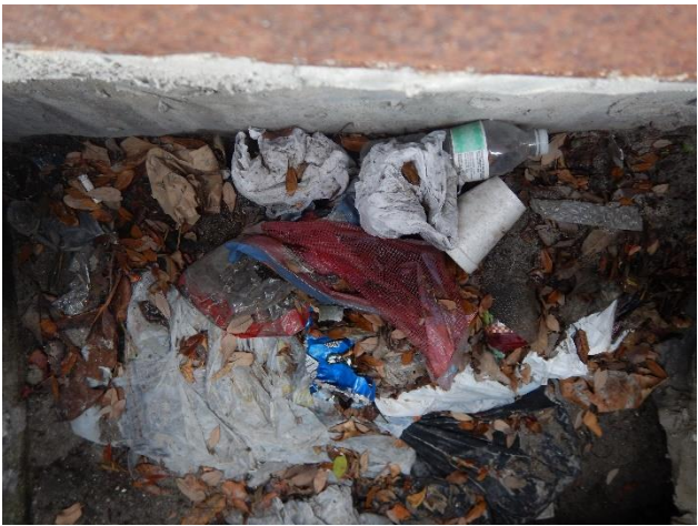
Photo 26 Impacted catch basin on Wingfield Street
