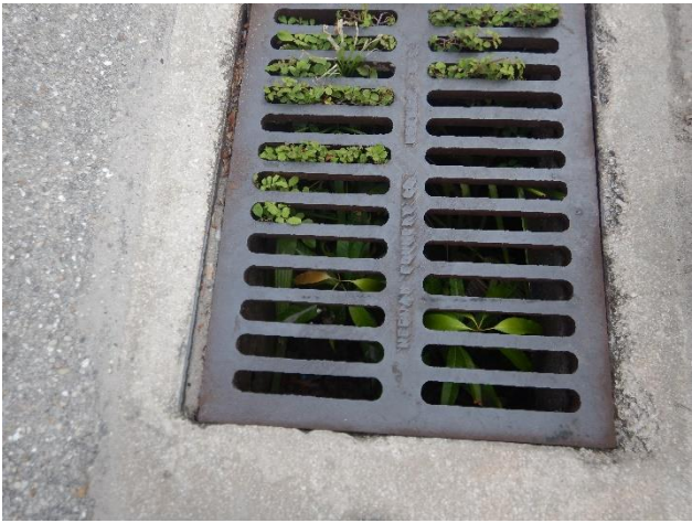
Photo 27 Impacted catch basin on Wingfield Street
