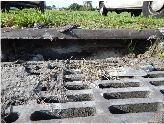
Photo 12 Table Enterprise Inc., debris washed to MS4
