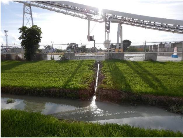
Photo 17 Illicit connection running directly form process
