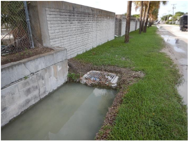
Photo 18 Illicit connection flowing to catch basin
