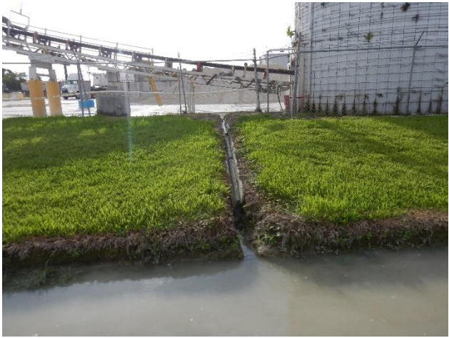
Photo 16 Illicit connection, no treatment prior to ditch
